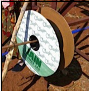
ROLLING OUT THE DRIP LINES
