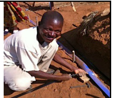
CONNECTING DRIP LINES TO SUB-MAIN
