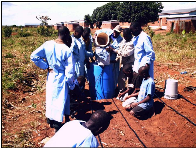
Installing Bucket Kits
